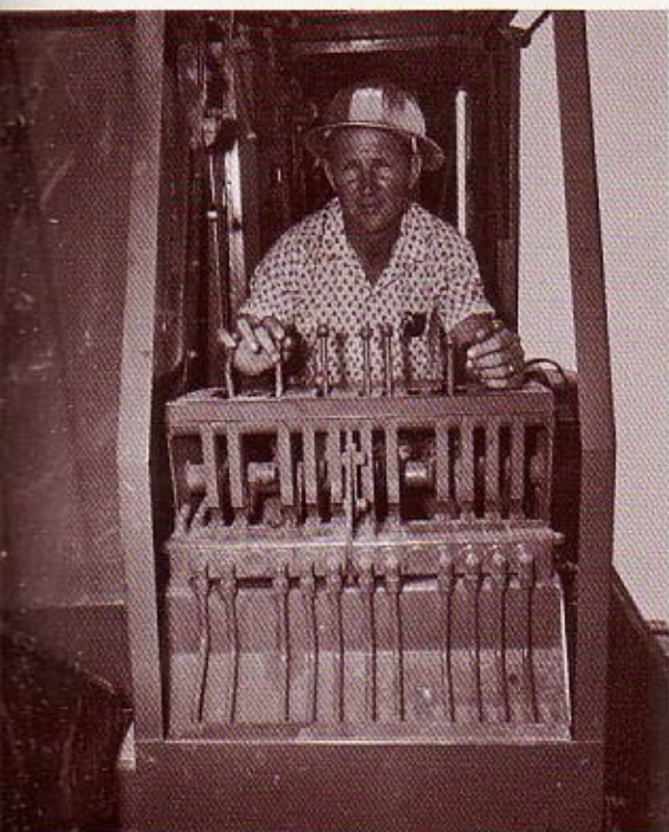
SPEED-O-MATIC CONTROL OF CARRIER. On all UC models, operator control of the major functions of the carrier is by Speed-o-Matic, the same full-power hydraulic system used to control all functions of the upper. This includes control of travel, steering, service brakes, parking brake release and transmission gear-shift on 4-axle models.
