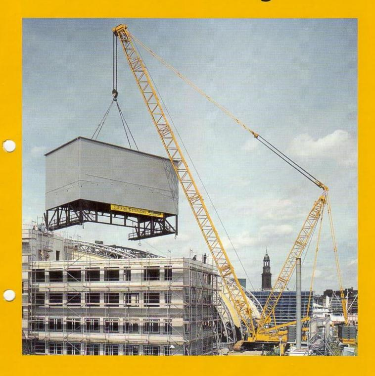
The Hamburg harbour has been the scene and skyline the musical "The Lion King", the top section of the stage for a spectacular lift performed by the teams of the crane tower had to be positioned. The 115 tons partially cased rental companies "Mobile Hubtechnik and Grohmann Attollo", both from Berlin. For the theater tent opposite to the piers, which is currently being transformed for
