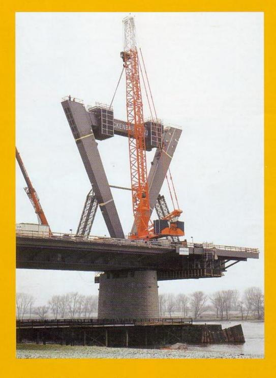
The major construction site "Rhine crossing A44" north of Düsseldorf was the first destination of the LR 1600/1, the crawler crane newly developed by Liebherr as "Pedestal Crane". The advantages of the new technology became evident during the positioning of colossal pylons on the foreland bridges: "The crane would nt have been in a position to work on crawlers
